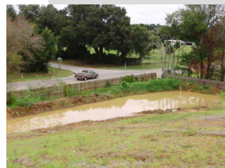
Before: Perimeter ditches constantly overflowed often causing flooding on the nearby roadway.
