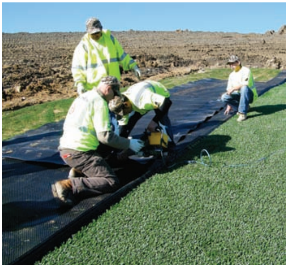
Installation had little impact on ongoing landfill operations.
