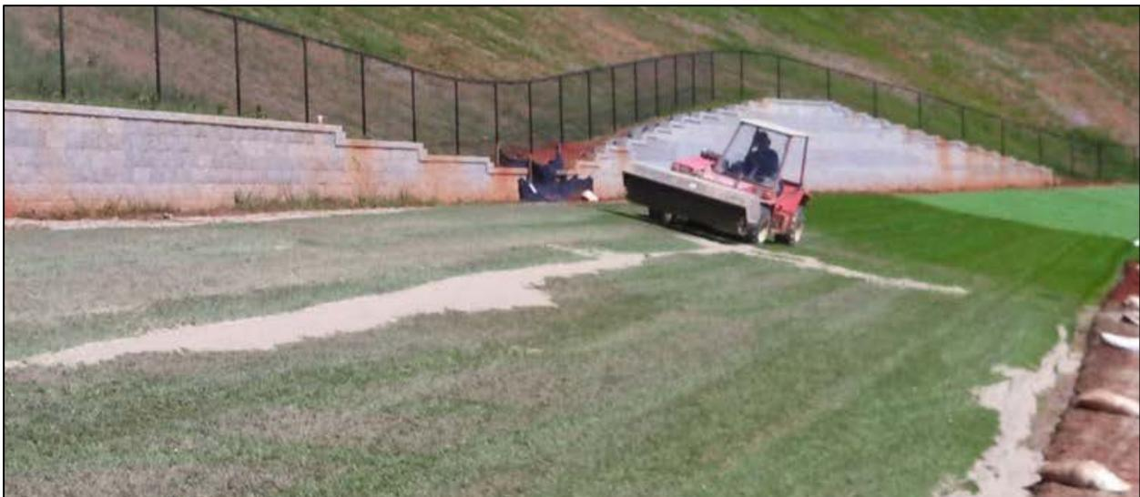
**Grooming the HydroBinder® material into the engineered turf.**
