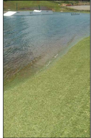
**HydroTurf protects against erosion from wave attacks.**
