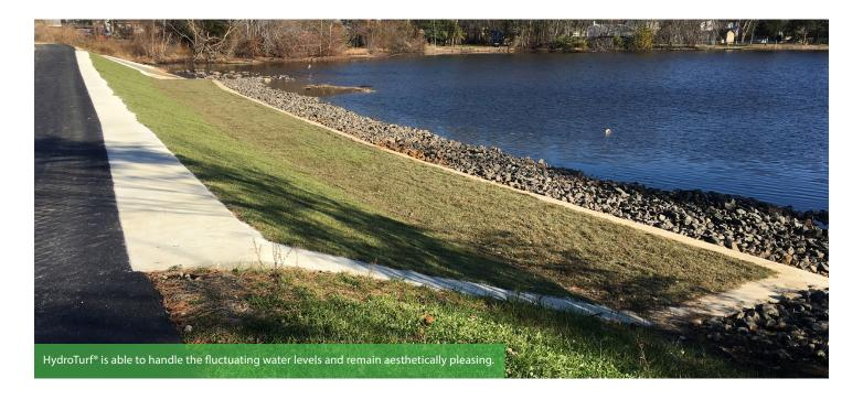
HydroTurf® was chosen for overtopping protection because it is a cost-effective, low-maintenance solution that will provide long-term armoring with the aesthetics of turf.
