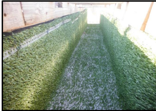
ClosureTurf® Installed in Channel (typical)
