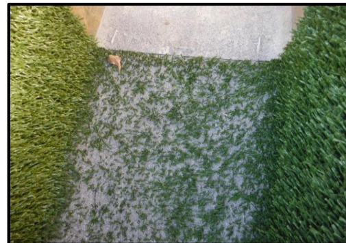
ClosureTurf® Installed (close-up)
