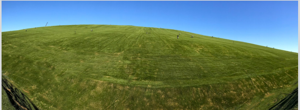
A view of the landfill showing the benchless slopes and the perimeter channel at the bottom.
