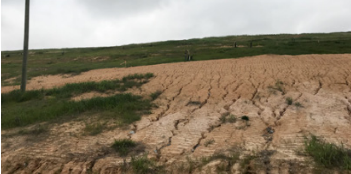
The site conditions prior to ClosureTurf installation.
