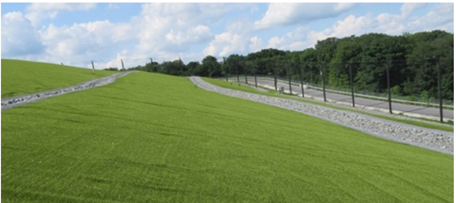
ClosureTurf® was easily integrated into the existing storm water management features.
