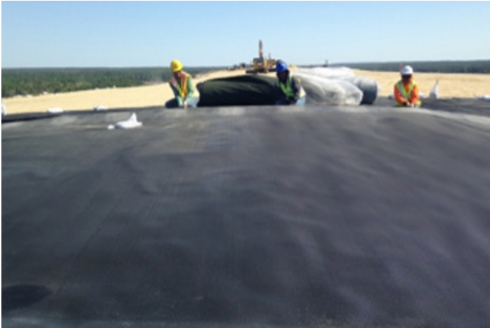
Installation of the Agru Super GripNet®.
