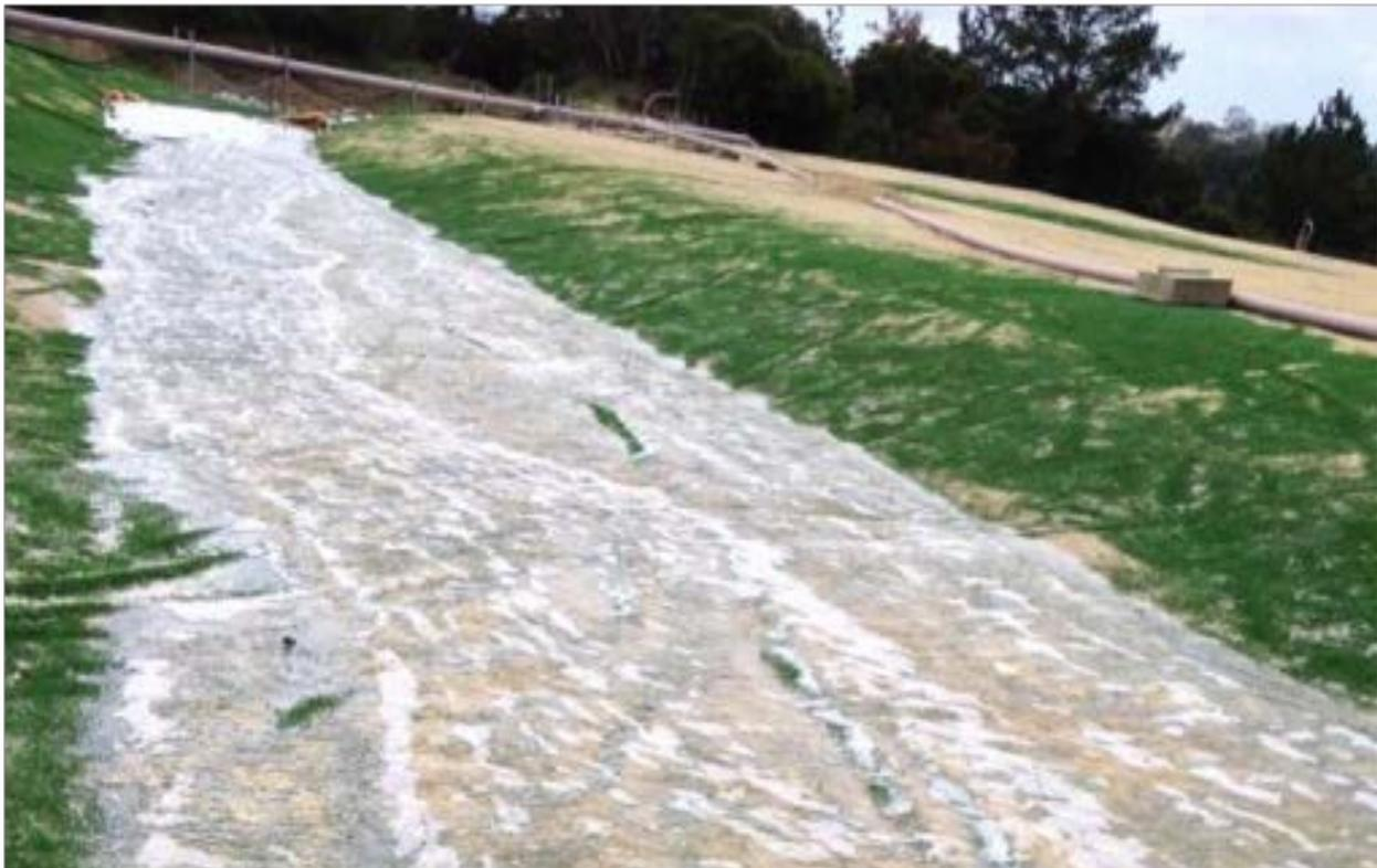
**The engineered turf and sand infill effectively filters surface water, providing clean runoff with very low turbidity.**
