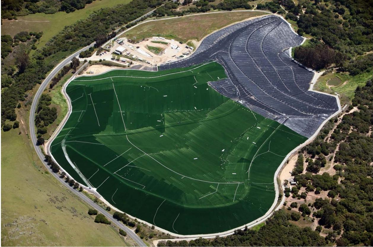
**Installation of engineered turf and geomembrane before sand infill is added.**
