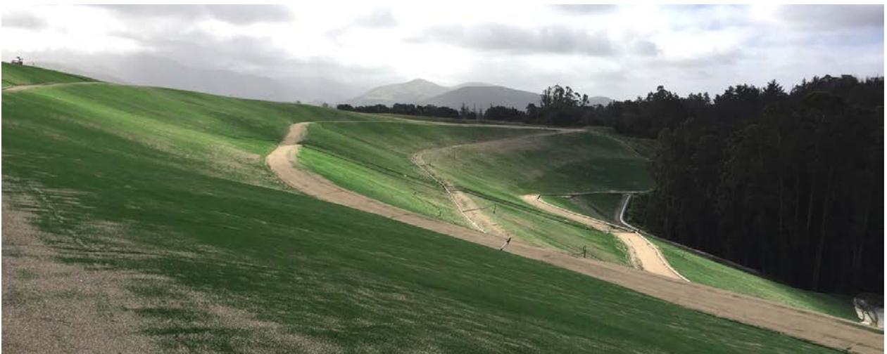
**Because some of the side slopes measure 2H:1V, Agru's Super Gripnet® membrane was used to provide a high shear strength.**
