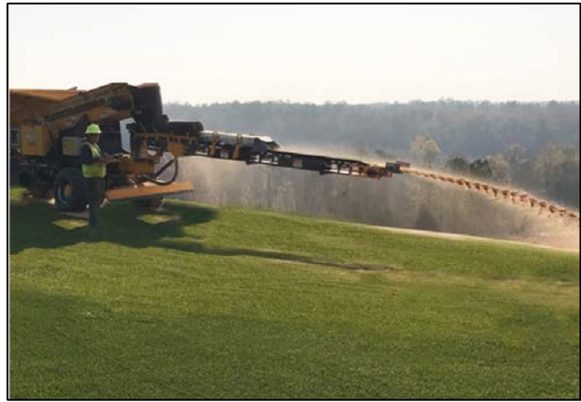
Sand being installed in the engineered synthetic turf.
