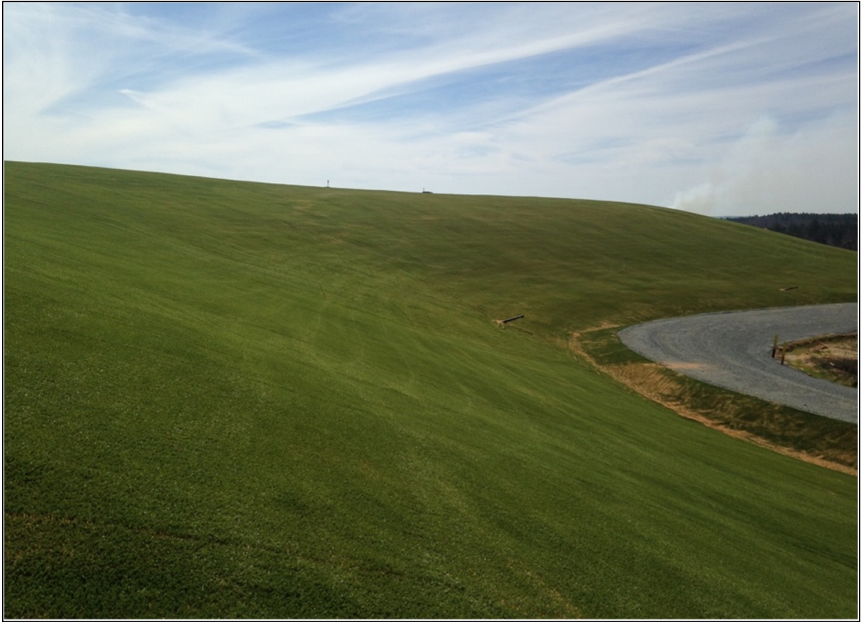
A view of one of the sideslopes at Baldwin County Landfill.
