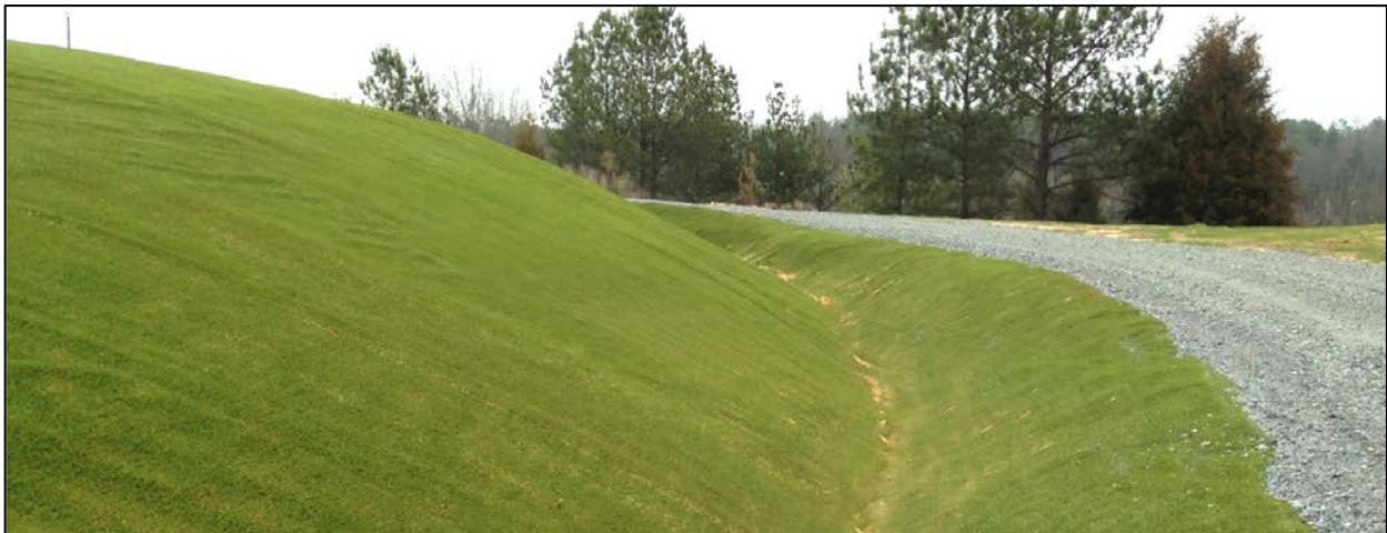
Perimeter channels are the only storm water mechanism needed to carry the water off site.
