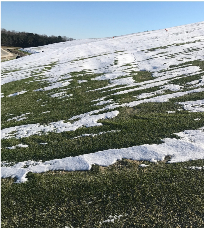
Snowfall on Accomack Landfill in 2017. ClosureTurf stands up to the harshest of conditions.
