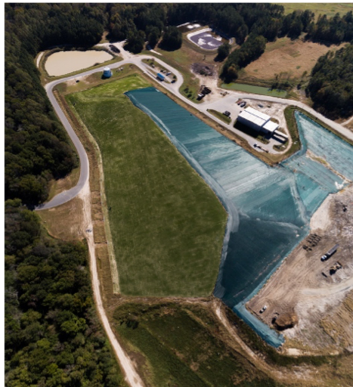
The use of ClosureTurf created an additional two feet of air space for waste disposal, providing a great economic benefit.
