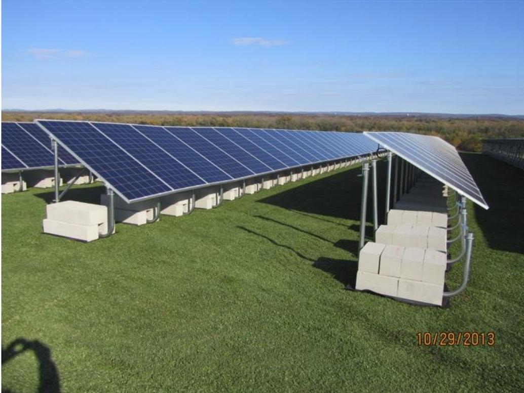
The superior drainage performance of the system mitigates runoff from the drip edge of the PV panels. The load-bearing characteristics of the ESTCS provide greater geotechnical stability to host the array and also allows for equipment and trucks to be used more liberally in construction of the array.
