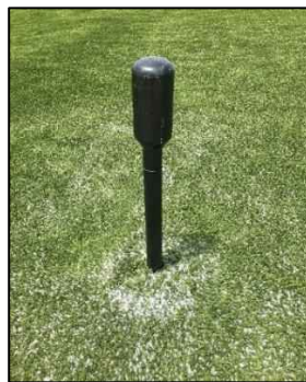
Figure 7-1. ClosureTurf Pressure Relief Valve (PRV) Installed in Field
