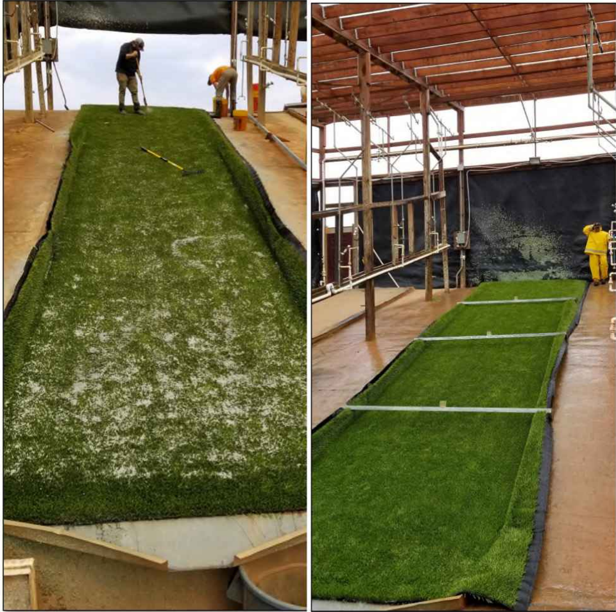
(a) Infill Installation
