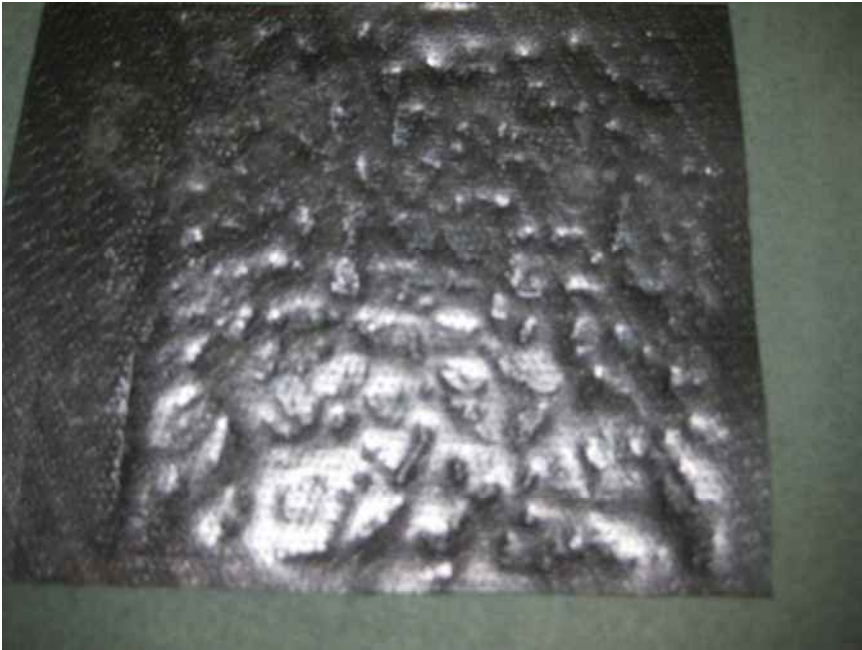
Figure 7. Deformed bottom surface of the geomembrane in contact with #57 stone after the completion of test. No punctures or holes observed.
