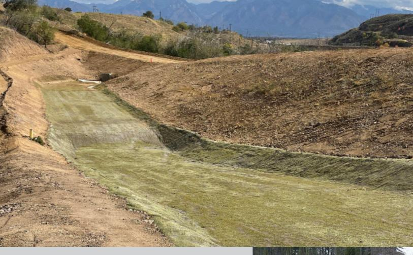
HydroTurf establishes long-term erosion control contributing to both environmental standards and ESG corporate benefits. The system is a Best Management Practice (BMP) that results in cleaner storm water runoff and reduces downstream maintenance of sediment ponds. HydroTurf is an impermeable solution that reduces contamination of surface and groundwater, resulting in reduced water treatment costs and site liability.
