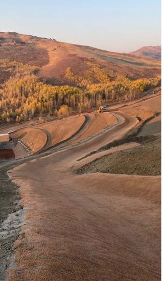
Used by mining operations throughout the U.S., HydroTurf® is a three-layered, engineered revetment system that was developed to meet the challenges of steep, high velocity channels and spillways on mining sites. It is both a flexible and impermeable hard armor technology which has lower construction and maintenance costs than traditional armoring products (i.e., concrete, rock riprap, articulated concrete block (ACB), and pipe).
