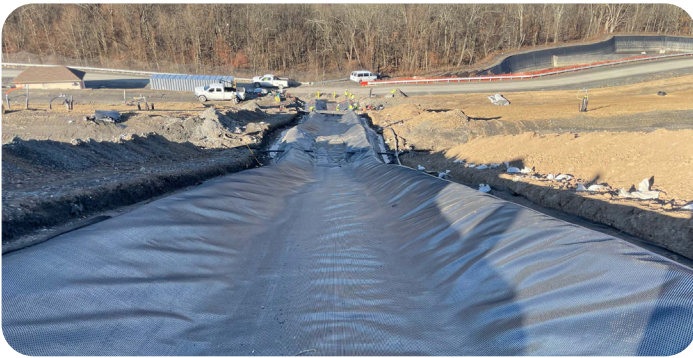
1. Geomembrane Deployment
