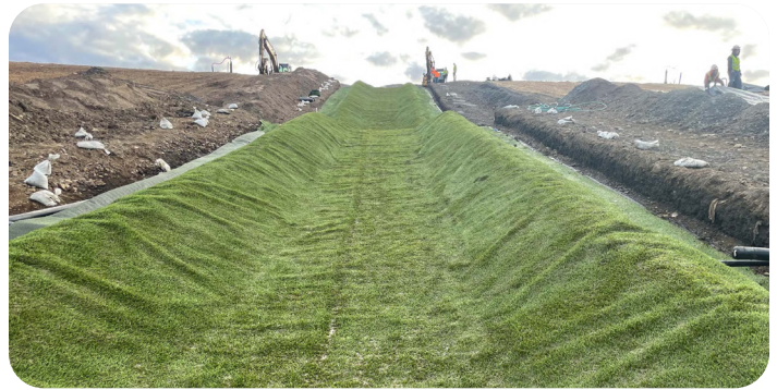
2. Engineered Synthetic Turf Deployment
