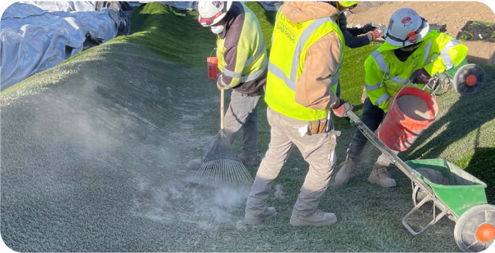
3. Spread HydroBinder® Infill
