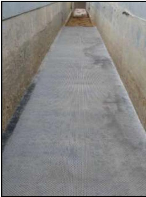
**Figure 3. Structured Geomembrane Installation**
