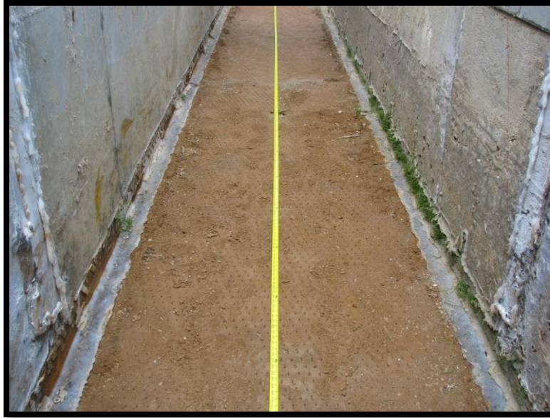
Figure 19: Soil Subgrade of Embankment after Testing of the CEST
