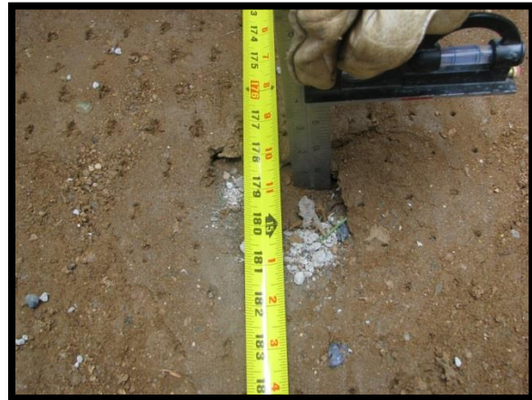
Figure 18: Soil Subgrade at Location of Intentional Hole after Testing
