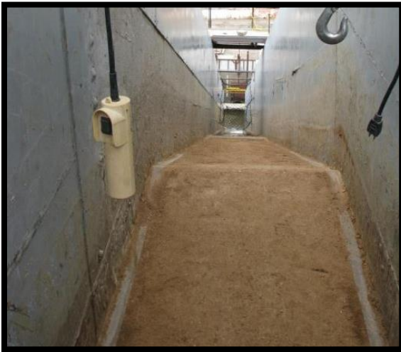
Figure 3 – Compacted Subgrade in Bottom of Flume
