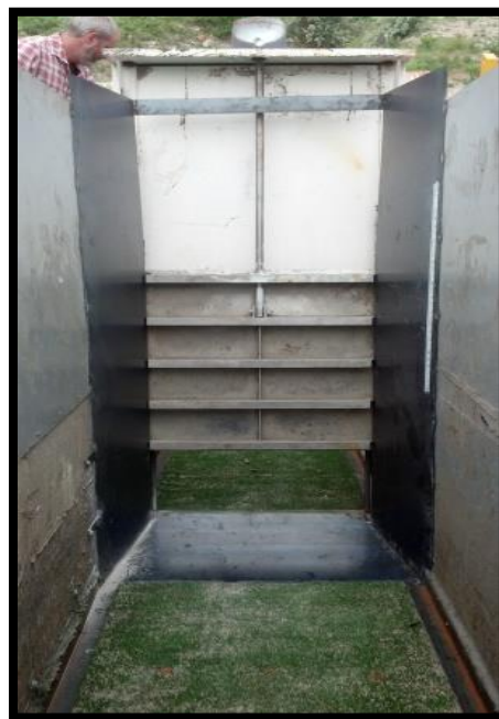
Figure 6: Vertical Sluice Gate Installed in the Overtopping Flume
