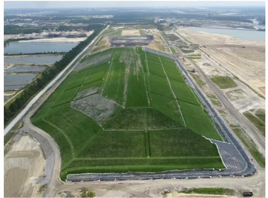
During Installation of Engineered Turf Cover (after Hurricane Dorian in 2019)
