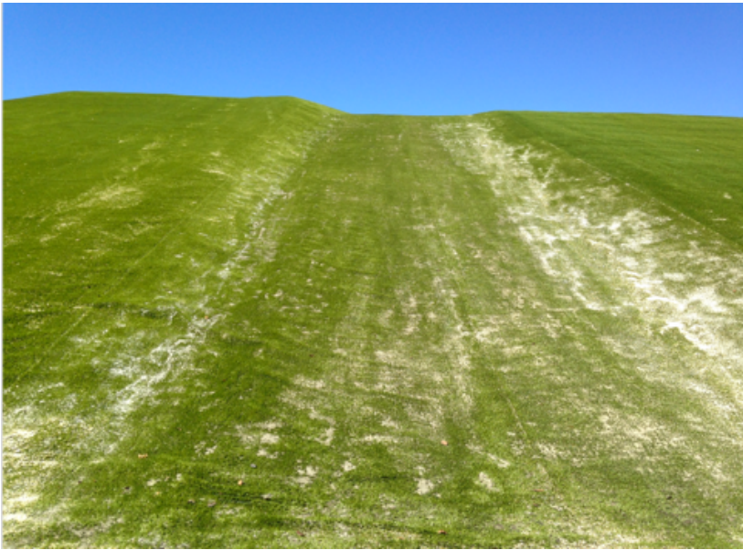
Engineered Turf Downchute with Cementitious Infill (October 2014)
