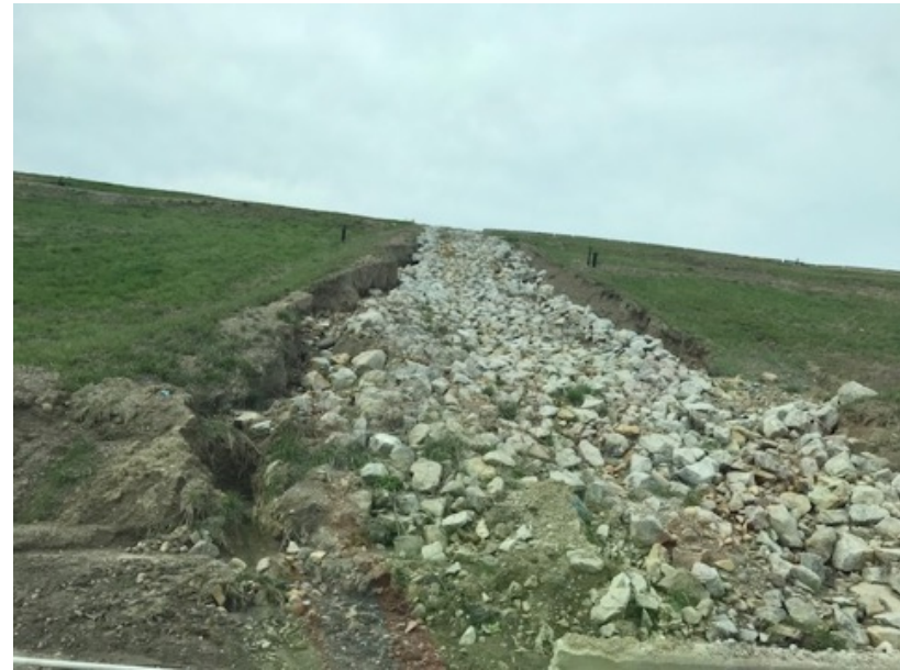
Typical Failure of a Rock Downchute (from another landfill site; shown as an example)
