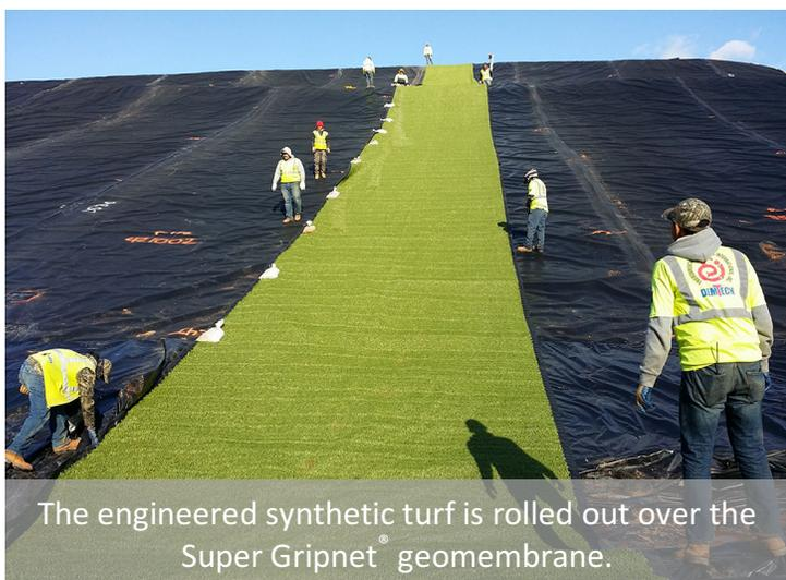
The engineered synthetic turf is rolled out over the Super Gripnet® geomembrane.
