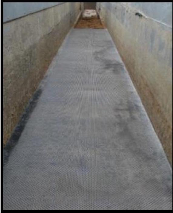
**Figure 3 – Installation of the Structured Geomembrane**
