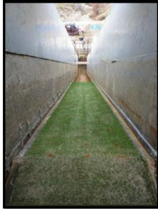
**Figure 4 – Completed Installation of the HydroTurf® System**
