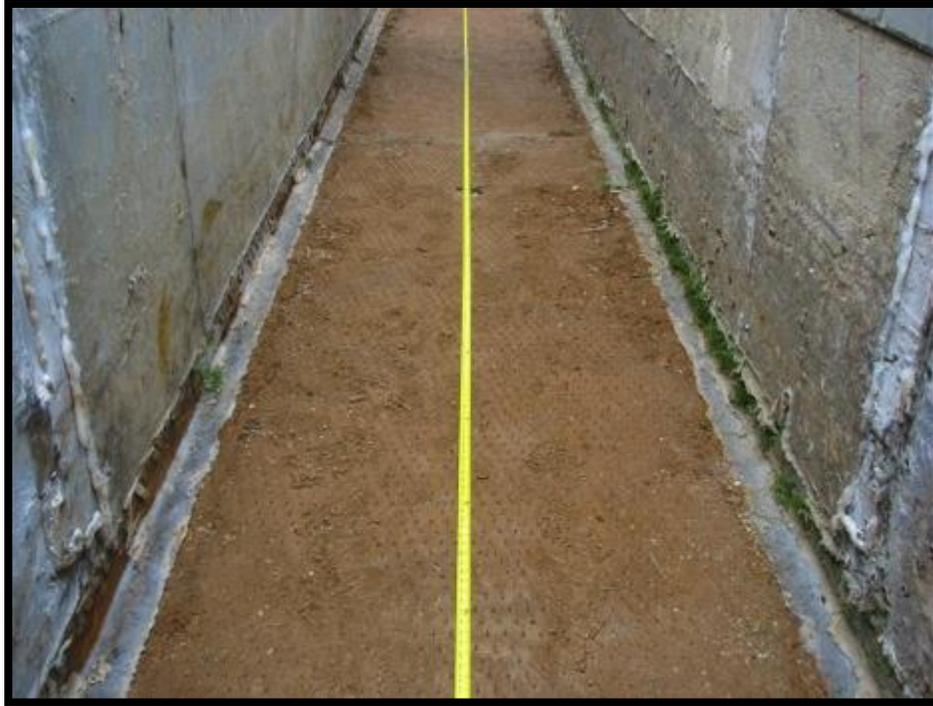
**Figure 19 – Condition of the Soil Subgrade
