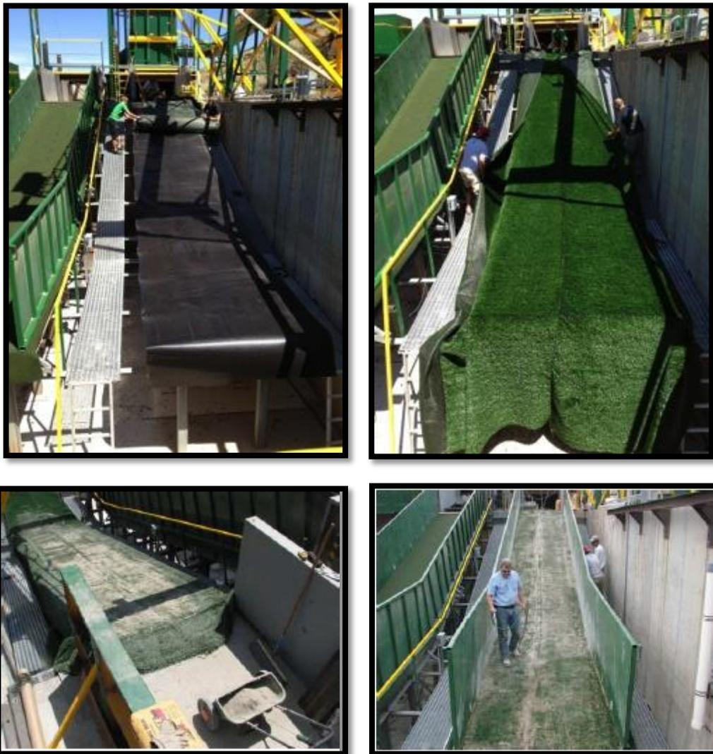
**Figure 22 – Installation of the HydroTurf® System**
