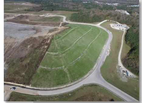
ClosureTurf® can be used for incremental closures as seen above in Berkeley's first four cells that met capacity.
