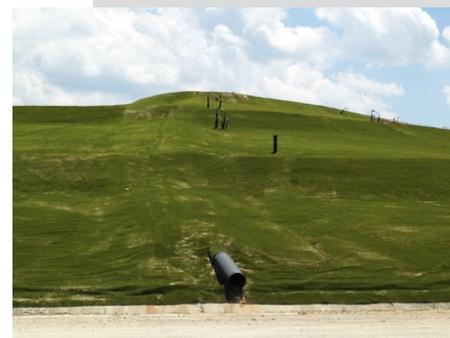
ClosureTurf® was easily implemented into Berkeley's conventional gas system.
