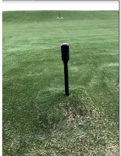
ClosureTurf can be incorporated into the landfill gas collection and control system (GCCS). Pressure Relief Valves were installed to relieve buildup in the case of unexpected landfill GCCS shutdowns.
