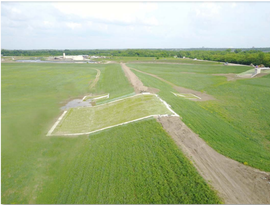
Aerial view of the upper and lower reservoirs.
